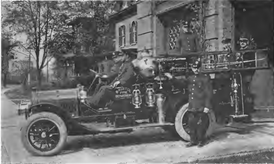
Combination Chemical and Hose Wagon for Bristol, Conn., Fire Department
